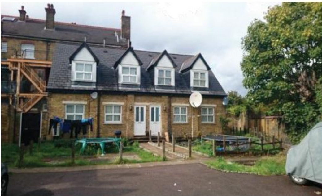
PH1- View of no.s 6 & 7 Priscilla Close and side access to no.8 Priscilla Close
